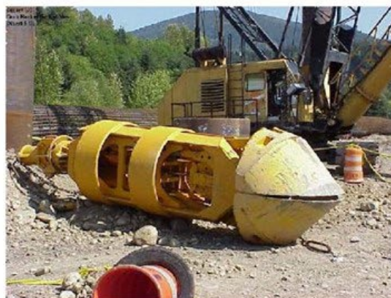
Clamshell Used for Removing Material from Drilled Shaft Casing
