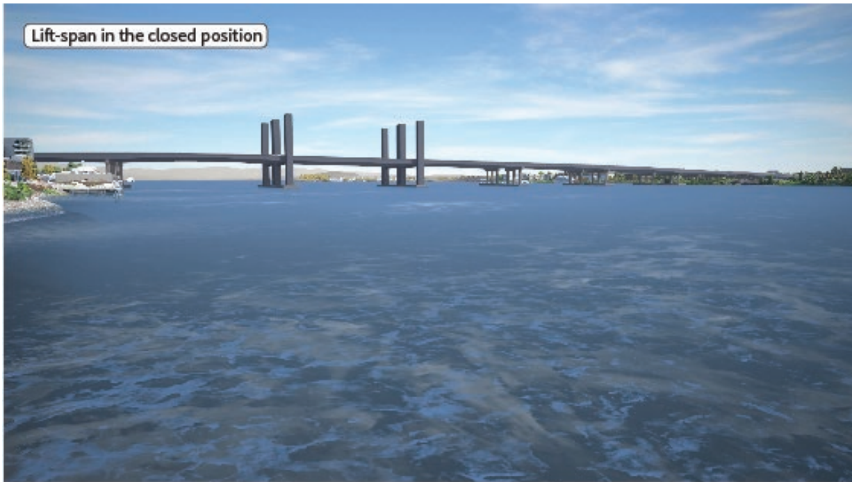
Figure 3-15. Example of Single-Level Movable-Span Girder Bridge in the Closed and Open Positions
