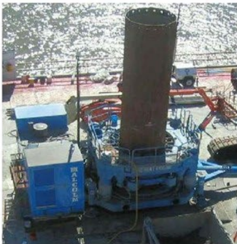
Typical Water-Based Drilled Shaft Installation
