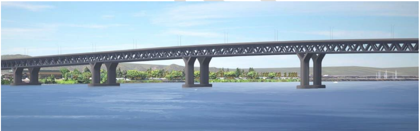
Figure 3-11. Example of a Double-Deck Fixed-Span Truss Bridge
