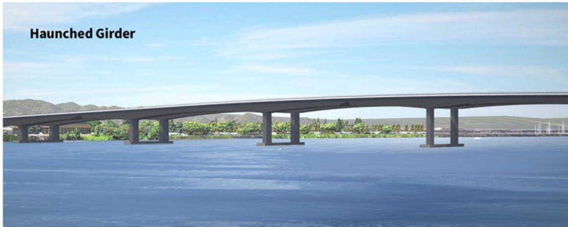
Figure 3-13. Examples of Single-Level Fixed-Span Bridge Types
