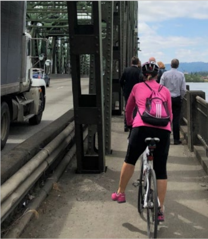
8 Figure 1-3. Bicycle and Pedestrian Path on the I-5 Interstate 9 Bridge
