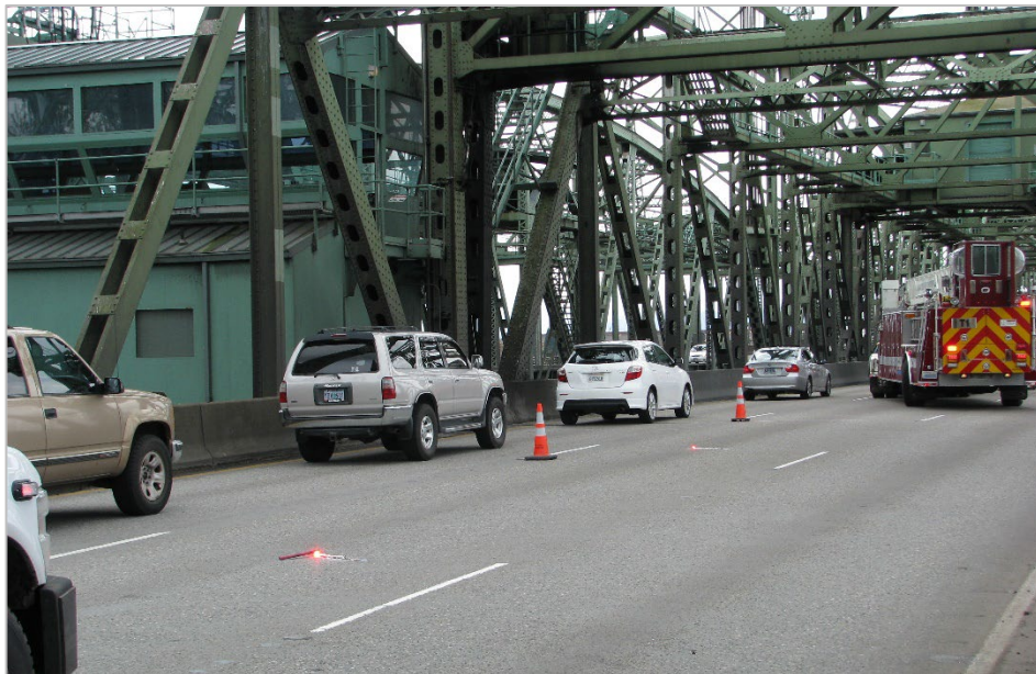
26 Figure 1-2. Crash Blocking the Interstate Bridge
