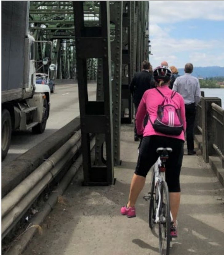
7 Figure 1-3. Bicycle and Pedestrian Path on the Interstate Bridge
