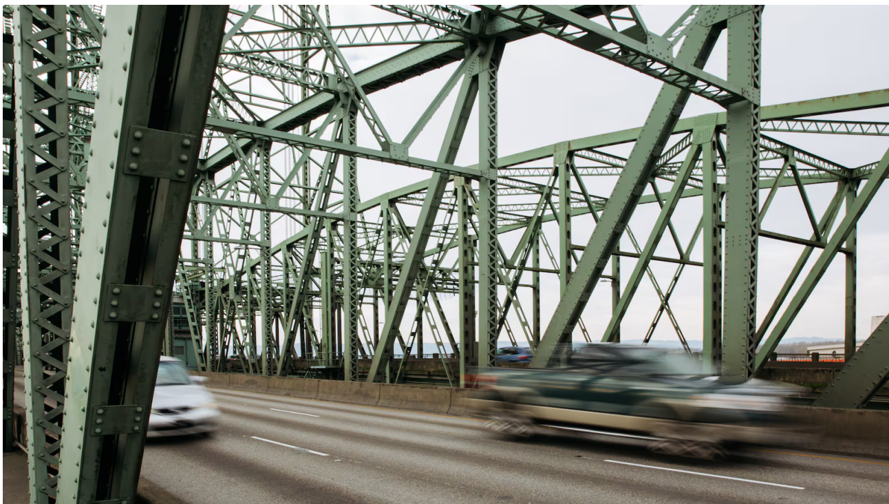
Traffic on the Interstate 5 Bridge. (Henry Cromett)
