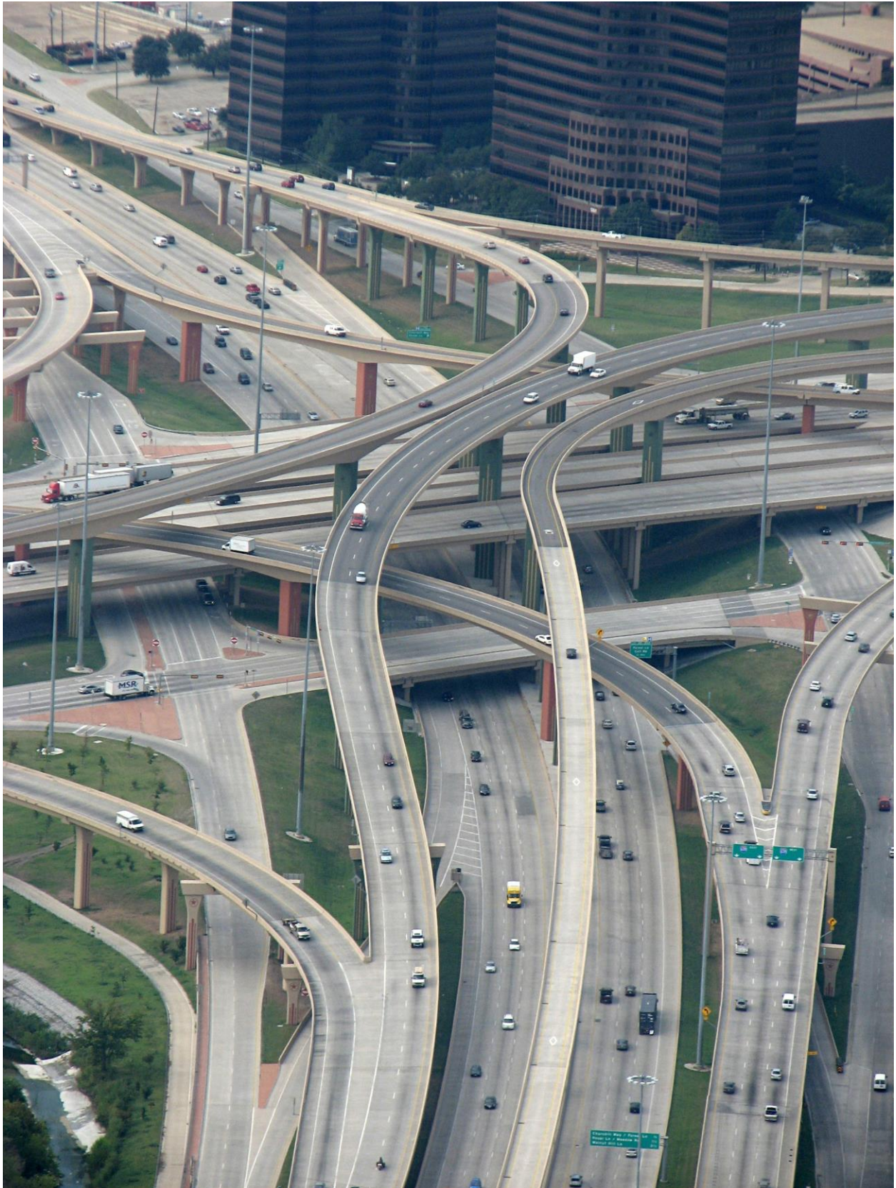
High Five Interchange at the intersection of I-635 and U.S. Route 75 in Dallas. Wikimedia
